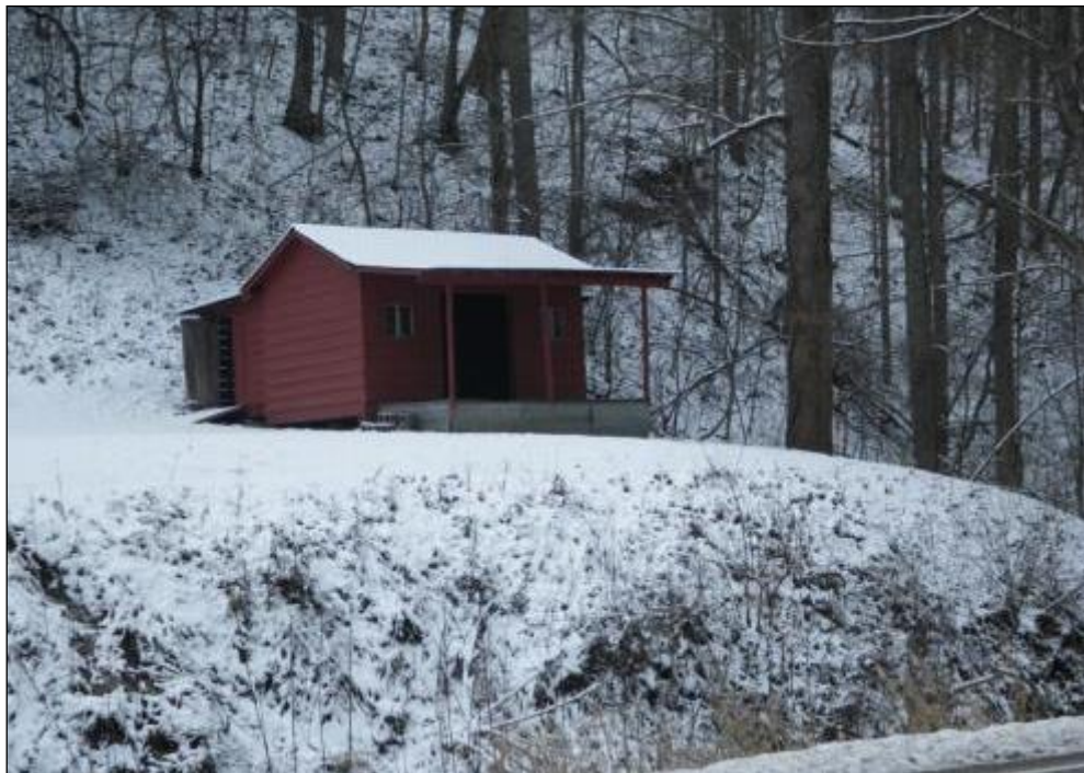
Figure 37. (R24) Structure near 6541 KY 632.
