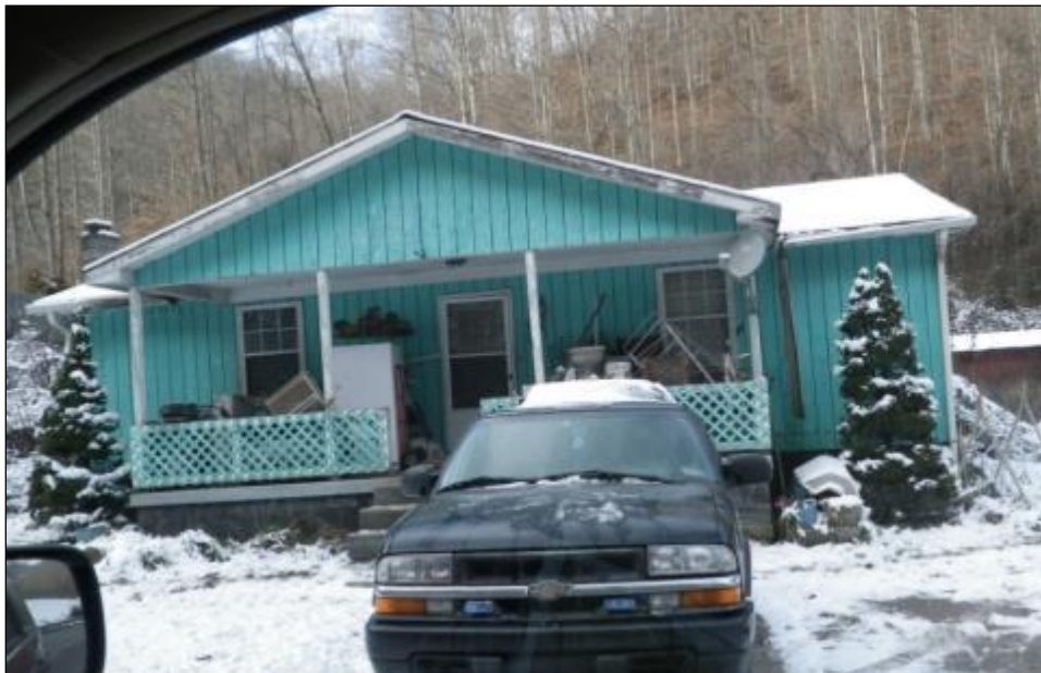
Figure 40. (R27) House located about 7828 KY 632.
