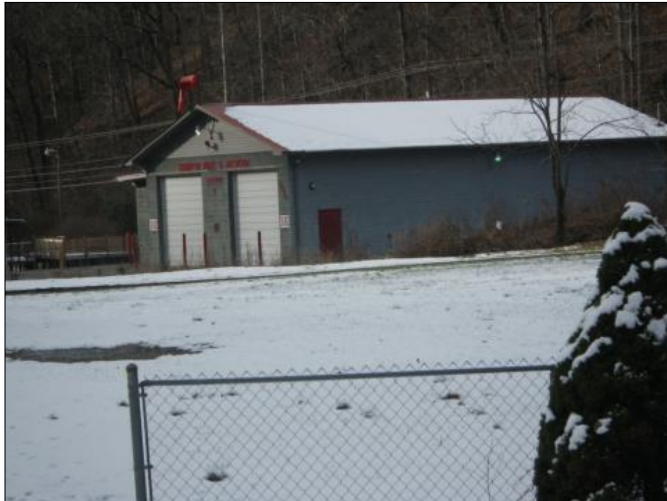
Figure 24. (R11) Kimper Fire and Rescue located at about 3822 KY 632.
