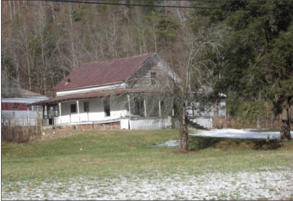
Figure 30. (R17) House located about 5794 KY 632.
