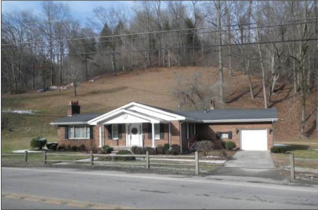
Figure 43. (R30) House at 12442 KY 632.
