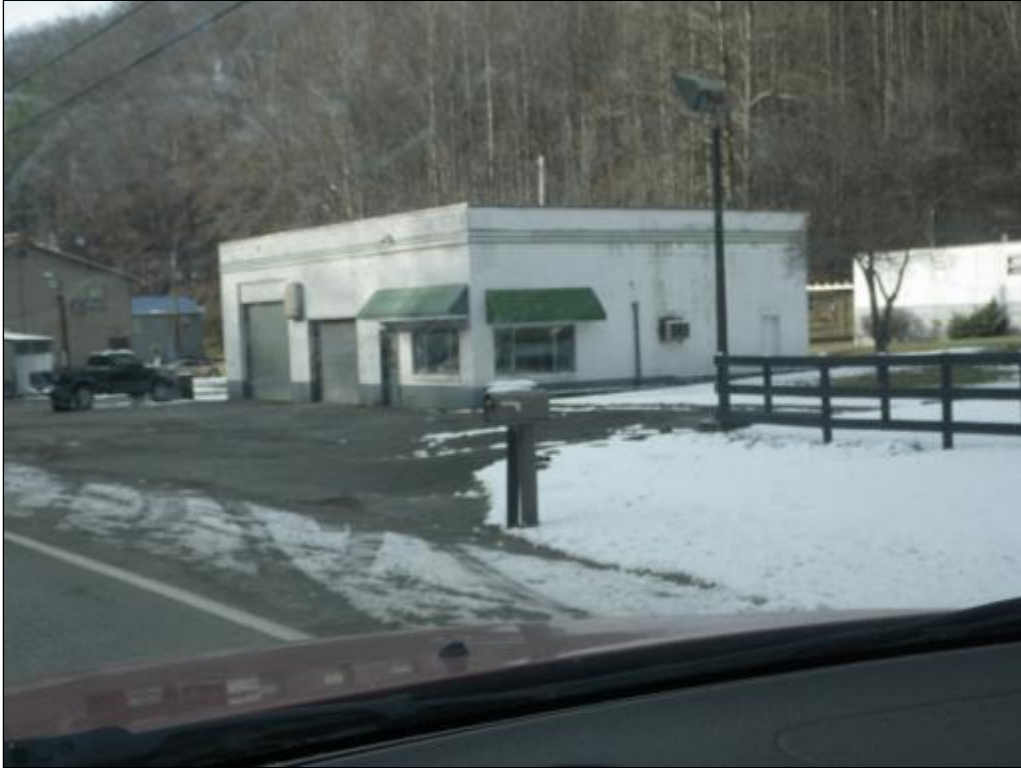
Figure 26. (R13) Service Station located at about 4548 KY 632.
