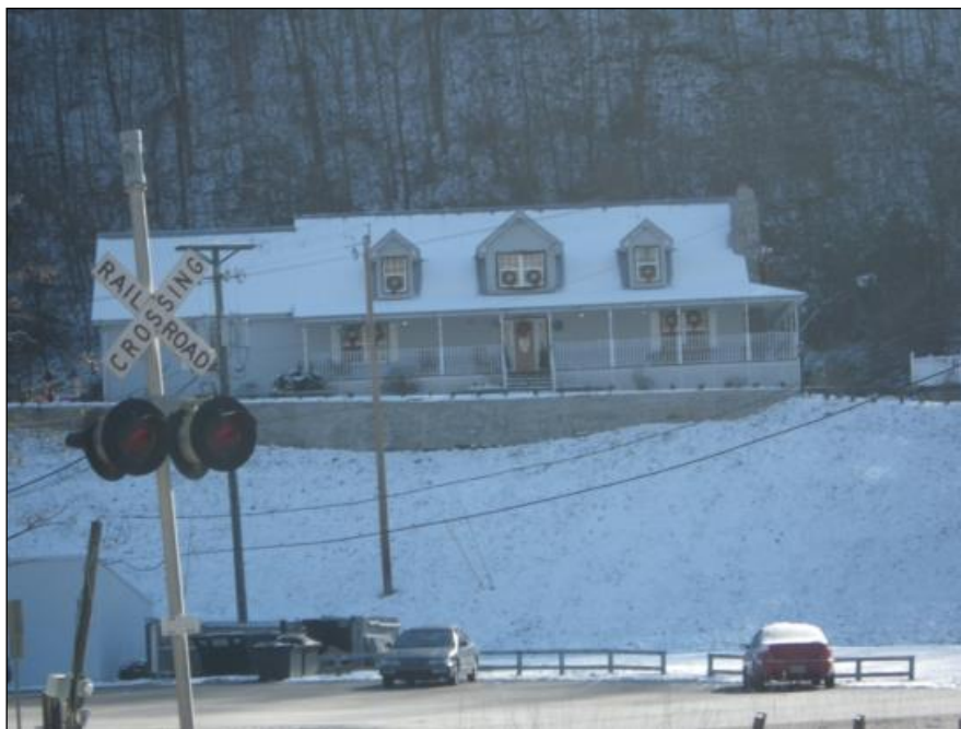
Figure 15. (R5) House, Intersection of KY 194 and KY 632.
