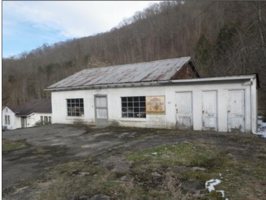
Figure 14. (R4) Store/service station located about 8972 KY194.
