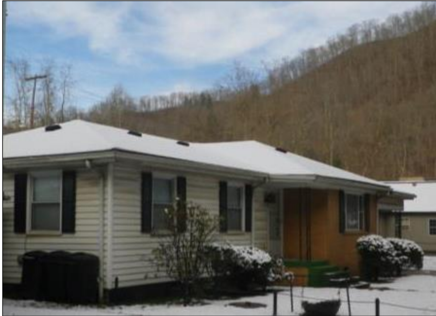
Figure 53. (R39) House at 13774 KY 632.
