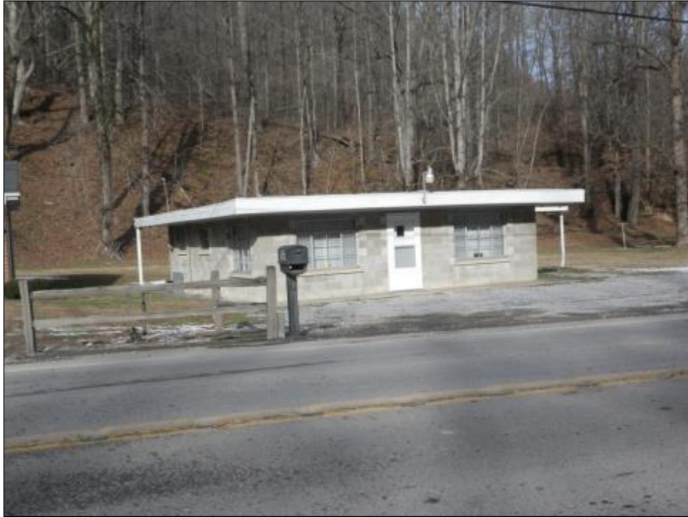
Figure 45. (R32) Building 12444 KY 632.
